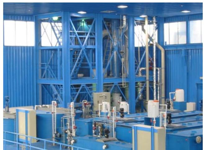
In the pre-purification step chemicals are added to precipitate arsenic and sulfate. The acid is then cooled and left for an appropriate ageing time. A flocculent is added and the solid content is allowed to flock (precipitate) in a clarifier.
